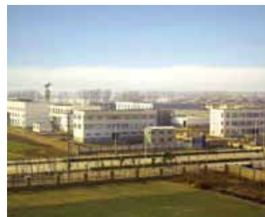
The new AEMC plant under construction
