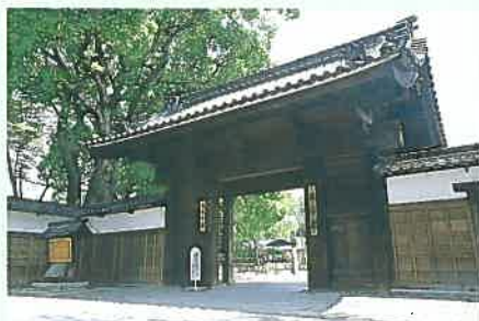
KUROMON This building reflects the architecture of the old samurai residence.
